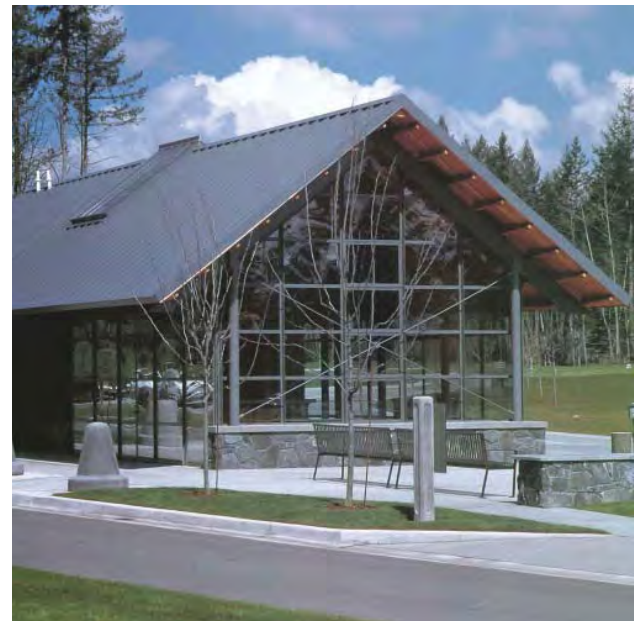
Provide quality materials and detailing
