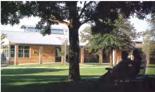
Buildings provide edges to streets and open space
