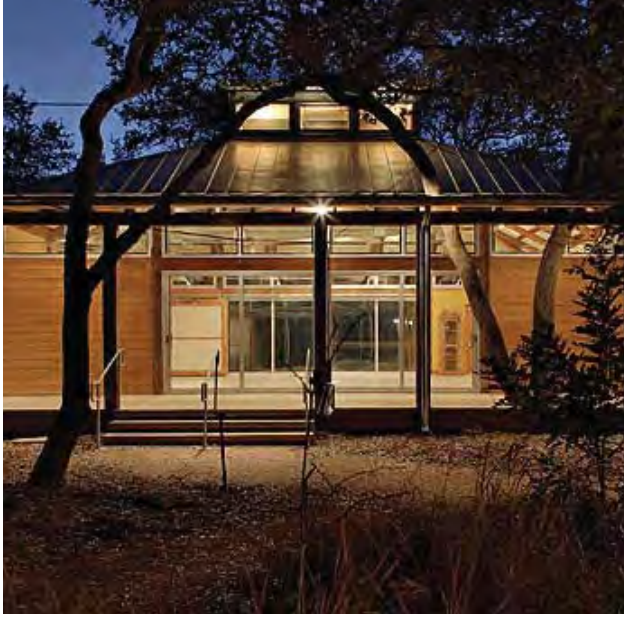
Lighting highlights architectural features
