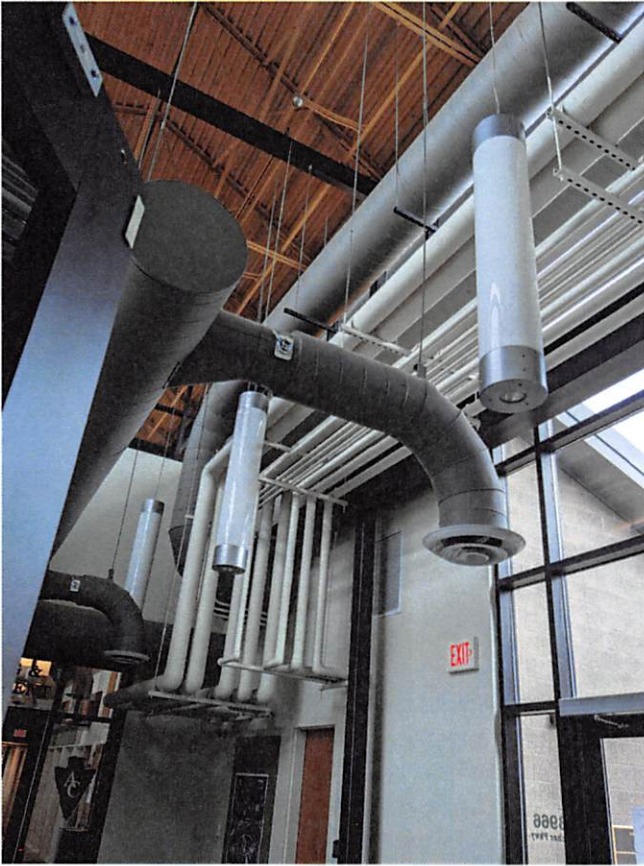
Existing duct work showing connection between coroners office and atrium into planning.
