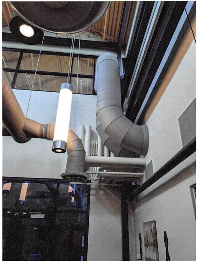
Existing duct work showing connection between coroners office and atrium into planning.
