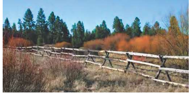
Buck and Rail Fence offers a transparent border and is wildlife friendly
