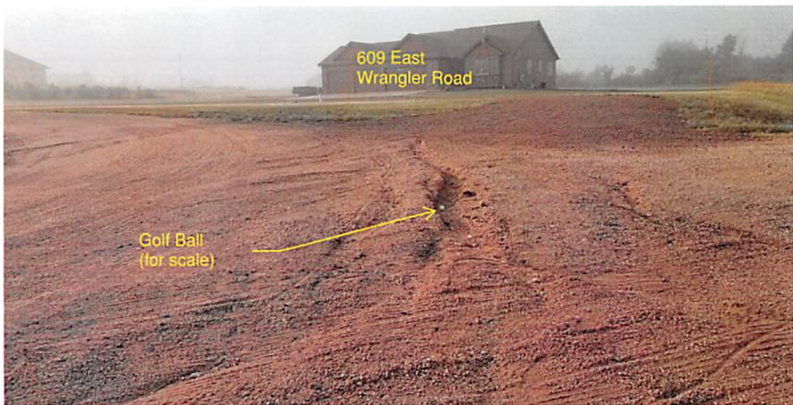
Figure 6 – Damage resulting from one rain event. 609 East Wrangler Road sheds water across both East Wrangler Road and Santa Fe Trail. While East Wrangler Road is a County Road, private maintenance is required. Allowing this condition to perpetuate creates a burden on the neighborhood that would presumably not be tolerated if maintenance were provided by Laramie County.
