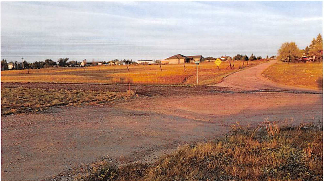
Figure 10 – Trench damage across East Wrangler Road still exists, despite recent maintenance. The road is maintained with private funds.
