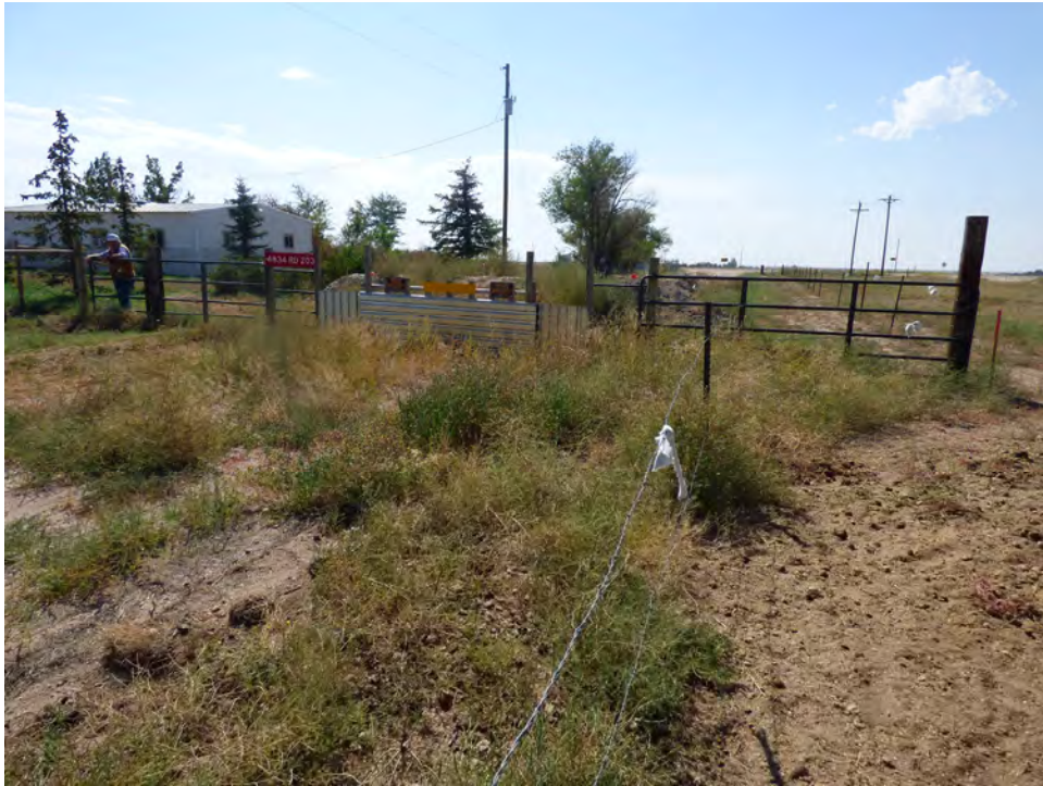
Dirt berm and fencing installed by owner
