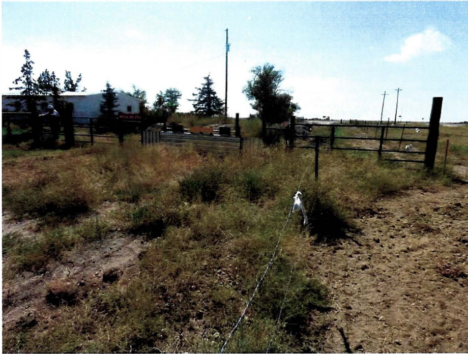
Dirt berm and fencing installed by owner
