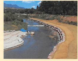
and bank stabilization measures including a proposed grouted boulder wall and single boulder drop structures for the emergency fix, working in close collaboration with the Utility.
