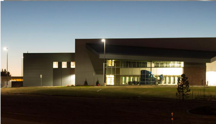
LARAMIE COUNTY COMMUNITY COLLEGE FLEX BUILDING AND SITE DESIGN WITH RYAN RIGG AS CIVIL ENGINEER WITH PREVIOUS FIRM
