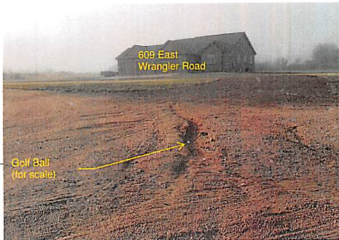
Road Damage on East Wrangler Road from one Rain Event
