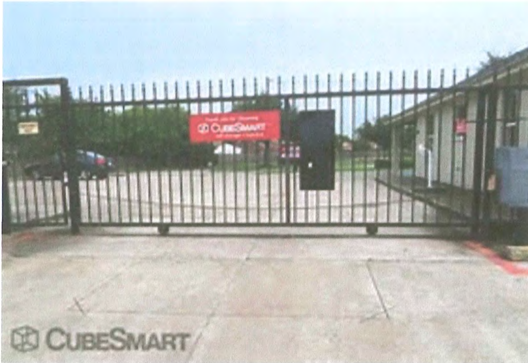
Secured with fencing and security cameras
